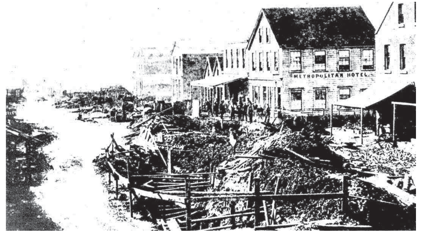
Circa 1865. Queen Street looking north at the collapse of the Ligar Canal
