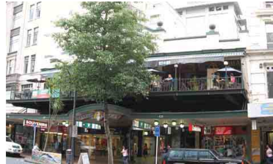
Sidewalk and elevated dining at Queens Arcade
