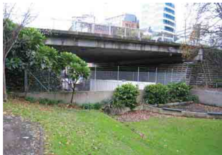
Flood detention area at the base of Myers Park and potential treatment wetland location
