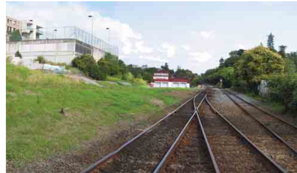
Looking west along the track and abandoned sidings to the railway sheds
